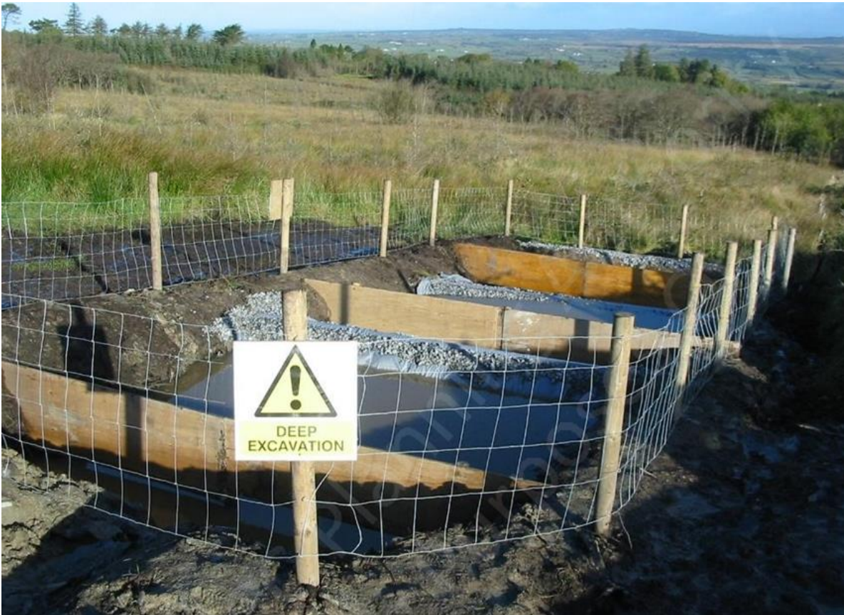
Plate 2-3: Example of a Three-Tiered Settlement Pond with Stone Filter
