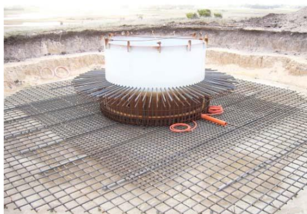
Plate 2-2: Steel reinforcement being added
