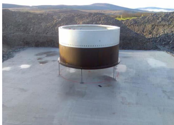
Plate 2-1: Levelled turbine tower “can”
